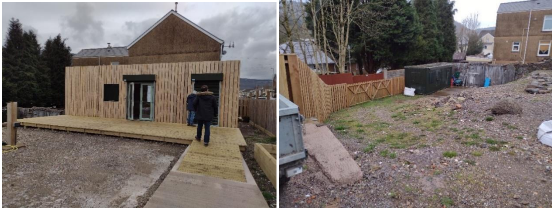
Figure 14: Treherbert CEA site - under development
